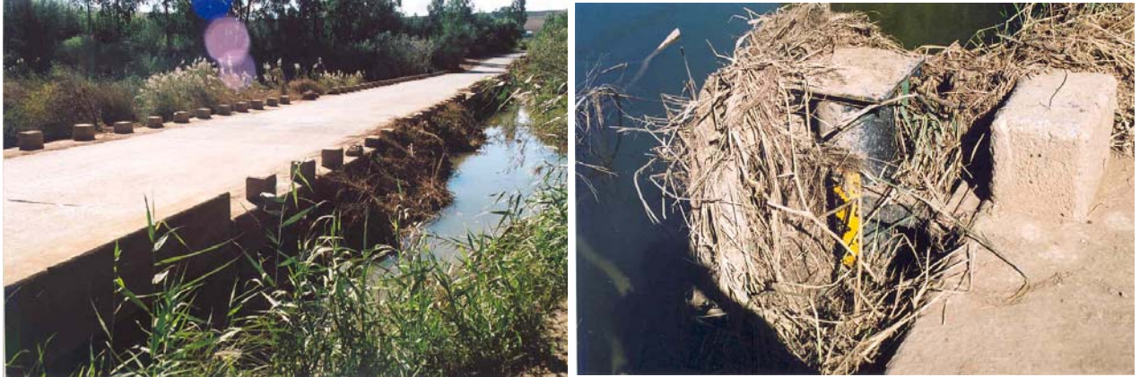
Figure 3.2 Reeds blocking the causeway below Lutzille 24 April 2005.
